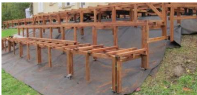
Figure 7 – structure support de platelage de terrasse
