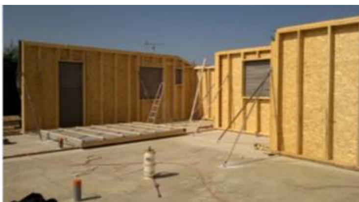
Figure 2 – Murs en ossature bois
